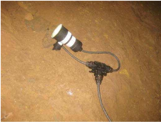
LED feature light and 'Techno' cable tee-off fitting. Photo: Daryl Carr
