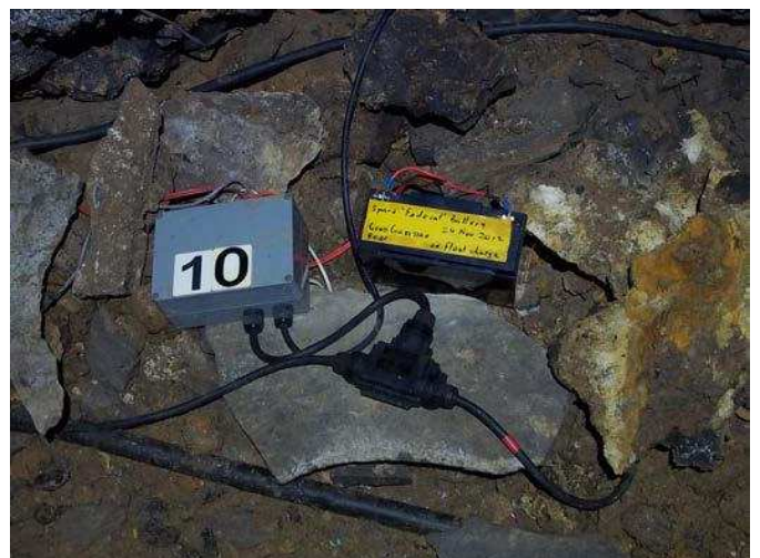
Control Box No. 10 with 12V sealed battery and supply from solar PV panel teed off from the 'bus' cable. Photo: Daryl Carr
