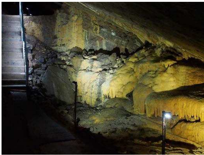
LED track lights mounted on existing wrought iron stanchions with LED feature light at base of left stanchion. Concrete steps illuminated by LED strip lights secured to guard wire below hand railing. Photo: Daryl Carr
